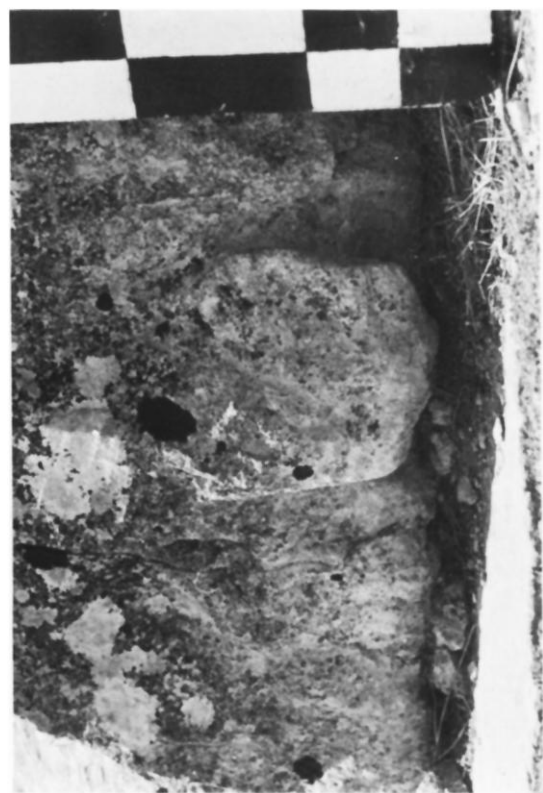
(a) Lifting boss at base of stylobate.
